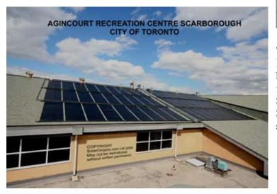
The Agincourt Recreational Centre uses 54 – 4' x 12' (241 sq. metres – 2592 sq. feet) of Techno-Solis solar collectors to heat the main pool at that facility. This system will be capable of to the main swimming pool a year. Over the projected lifetime of the solar system (20 years), it could displace the use of \$325,000 worth of natural gas and prevent the production of over 520 tonnes of green house gases.
